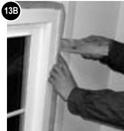
**IMPORTANT: Do not screw through the sill; use trim or structural adhesive to secure.**
